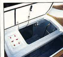
Top: twin Racor pre-filters with a changeover valve also come equipped with a vacuum gauge; not only can you switch filters with the engines running if dirty fuels strikes, but you can see when a blockage is looming long before it causes a problem. Above: the lazaret entrance into the engine room has a handy-placed fuel management panel located alongside.
