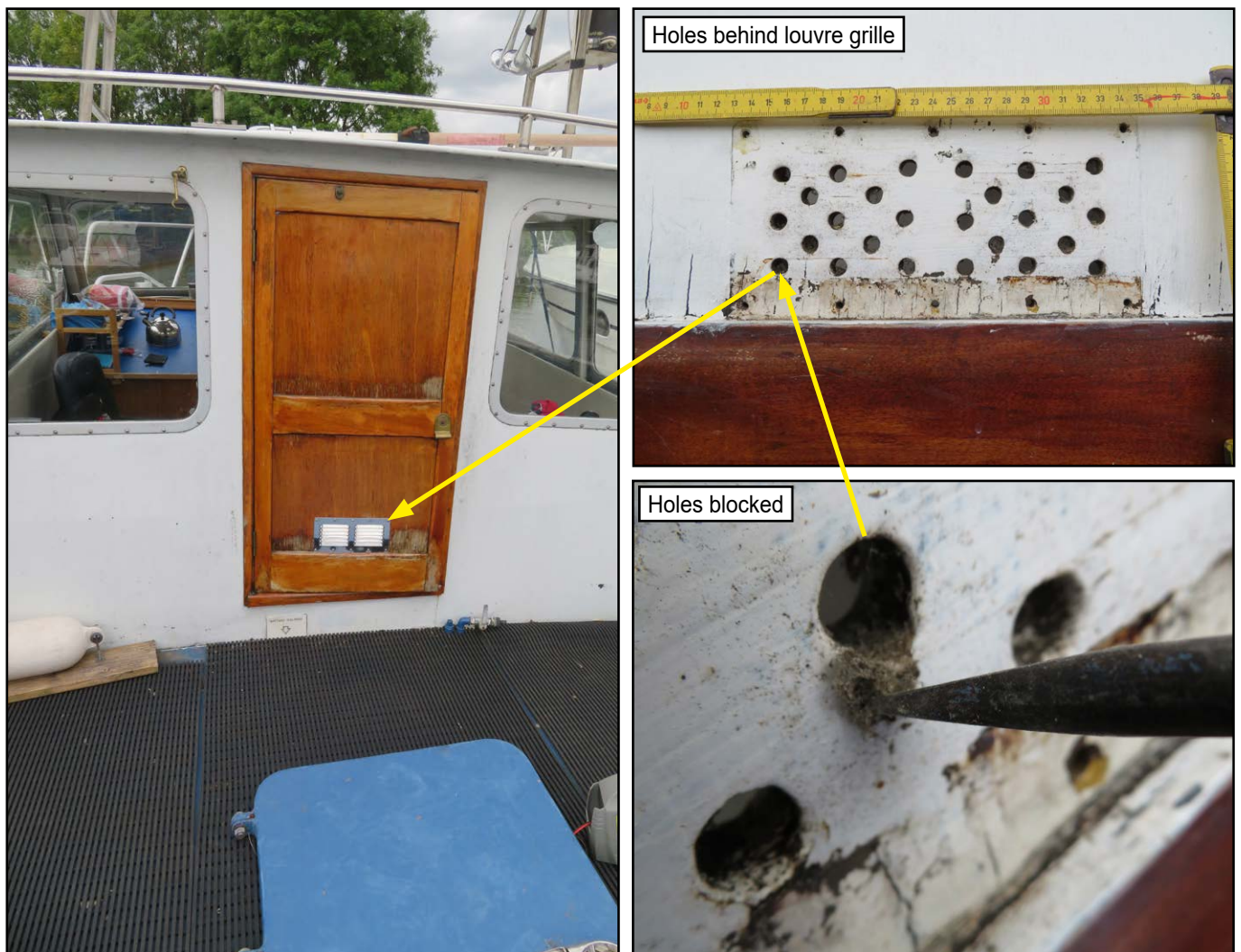
Figure 6: Wheelhouse door louvre vent
