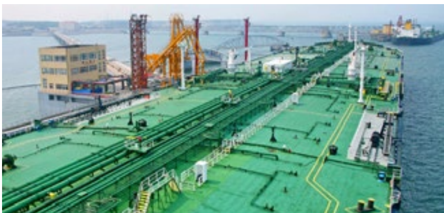
Crude oil tankers must protect their cargo tanks against corrosion. Corrosion-resistant steels have shown to be a viable and attractive alternative to protective coatings
