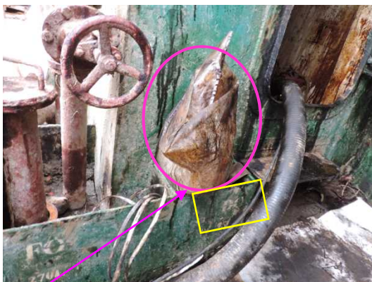
① Deck house side of port-stern part
