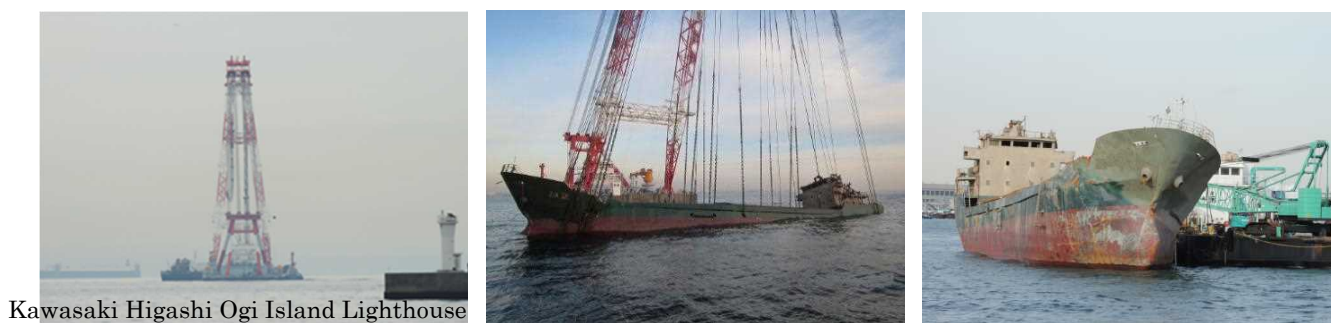
Raising work by crane vessel
