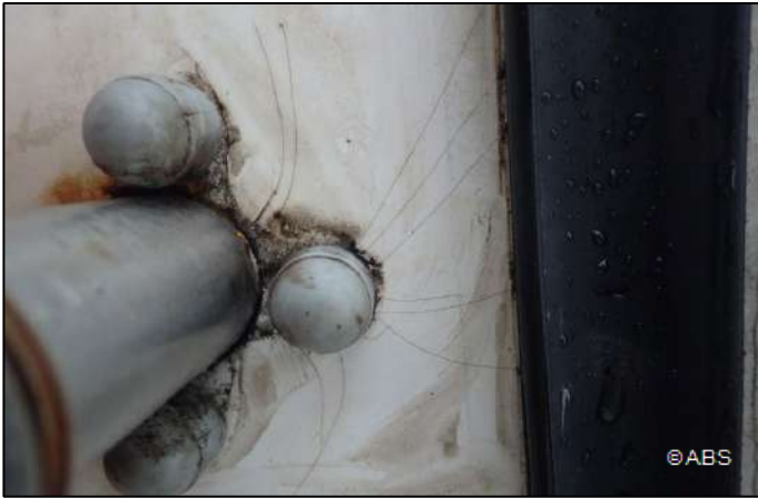
Free fall lifeboat door cracked around the hinge
