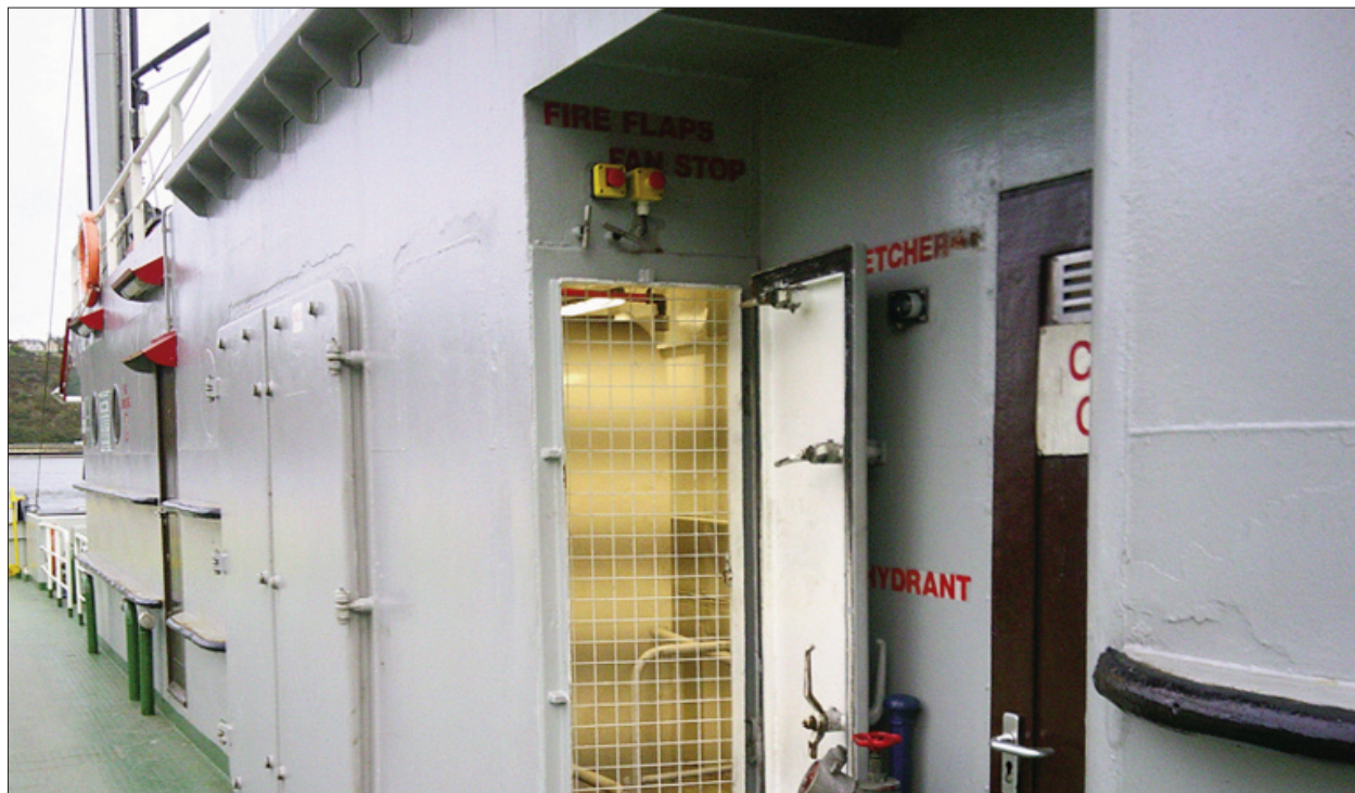
Appendix 7.5 Photograph No. 2 - Starboard Machinery Space Access Door
