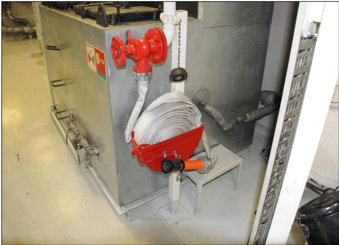
Figure 25: Standard jet pipe / hydrant system
