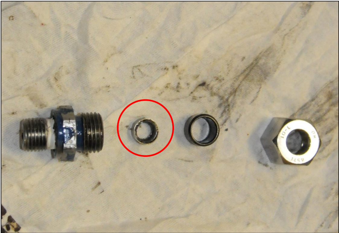
Figure 14: Fitting with broken-off piece of pipe
