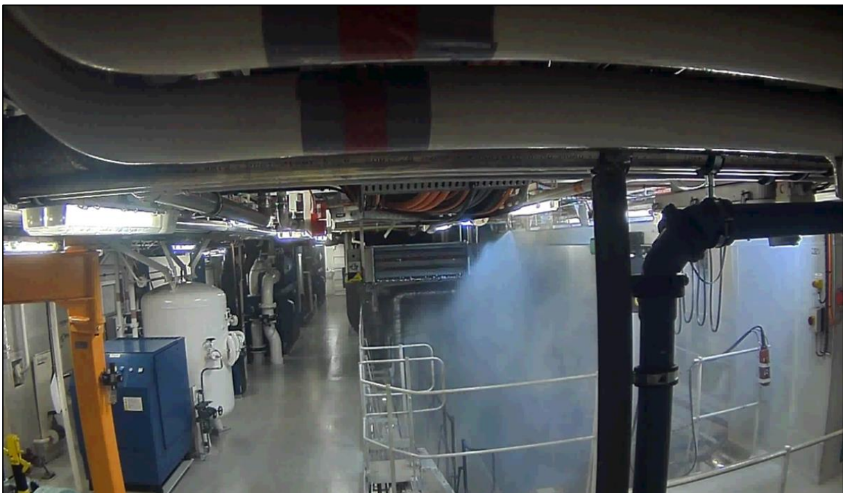
Figure 5: Object protection system triggered above ME 3 10
