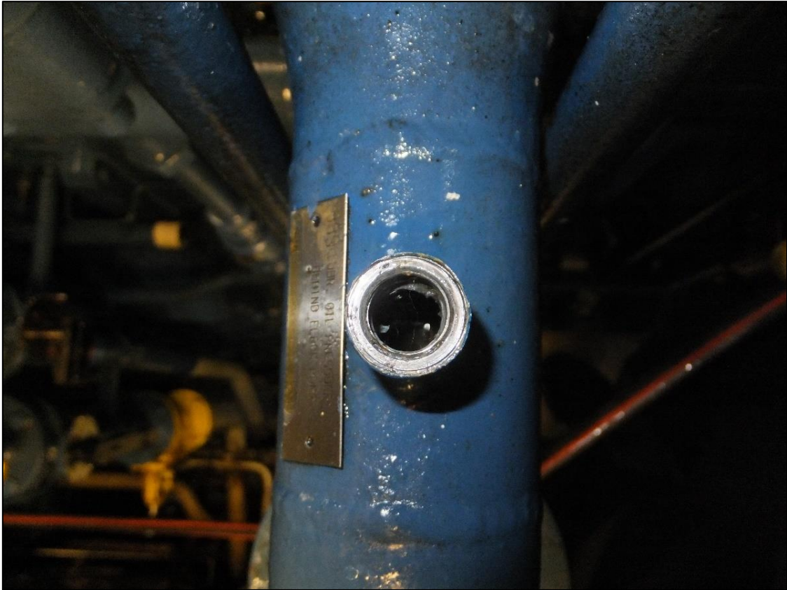
Figure 10: Open connecting piece (without double nipple)
