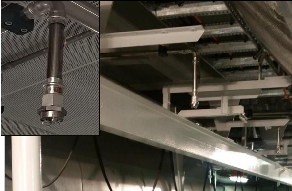
Figure 29: Object protection assembly above engine
