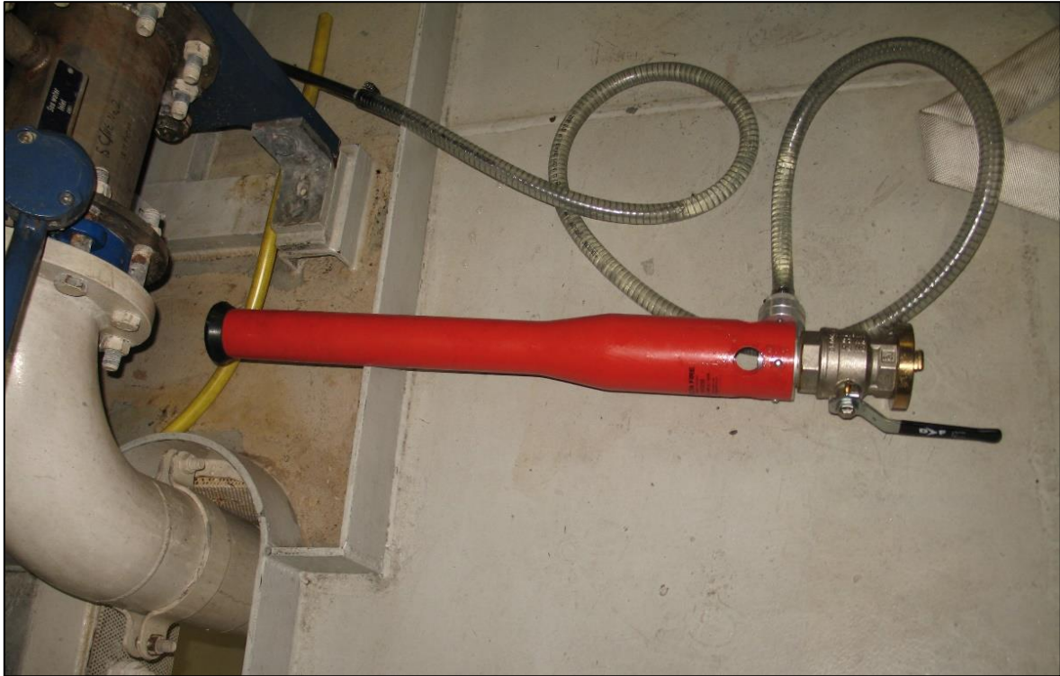
Figure 27: Mobile low-expansion foam pipe with integrated inductor
