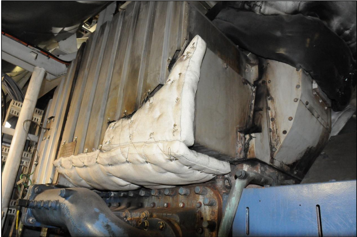
Figure 39: Additional insulating measures
