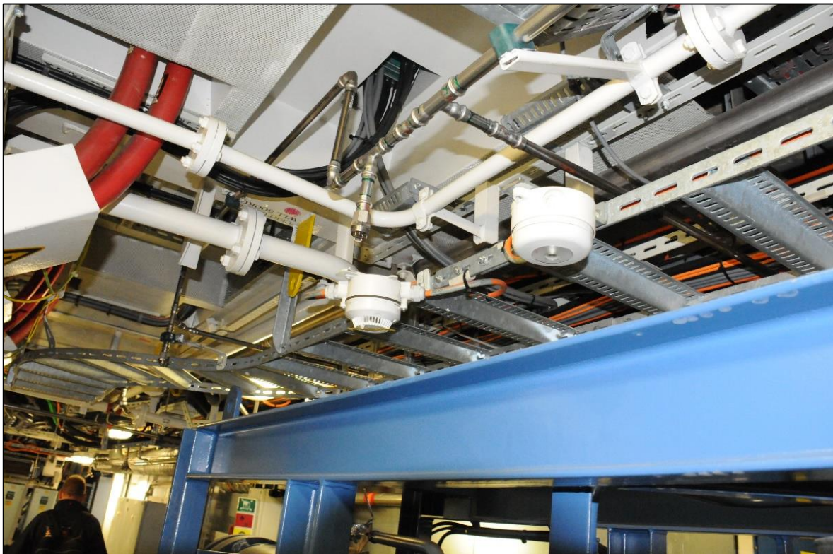
Figure 28: Object protection system
