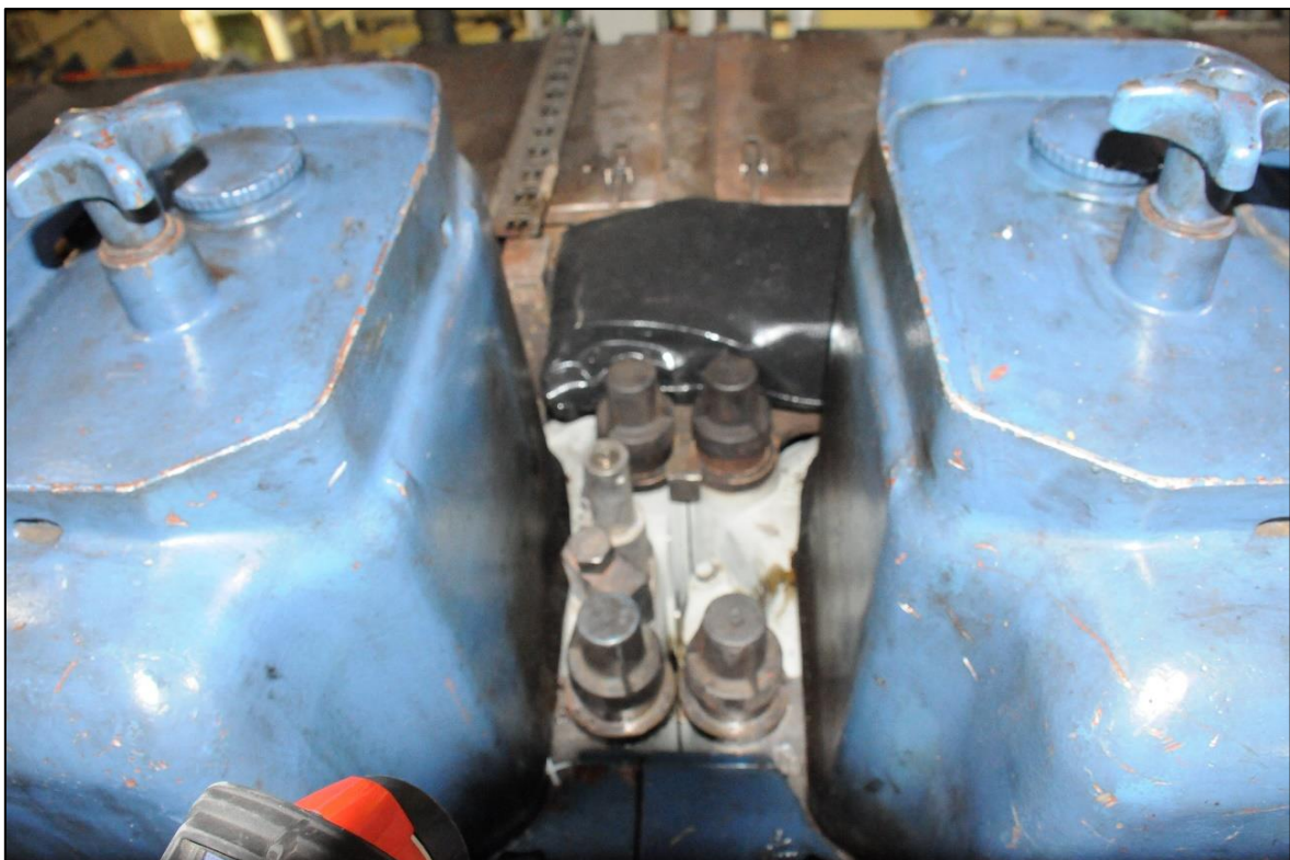
Figure 42: Insulation between cylinder station and exhaust pipe
