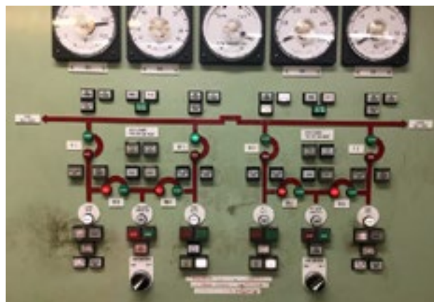
Figure 1: Main switchboard
