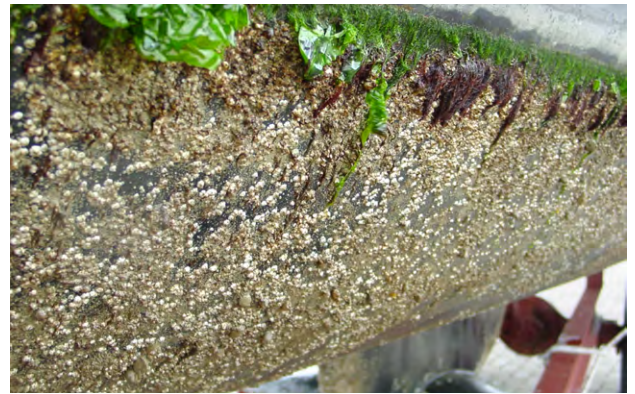
Macrofouling on a motor vessel
