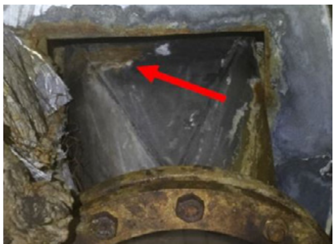
Temporary repairs on hull performed by diver on another vessel
