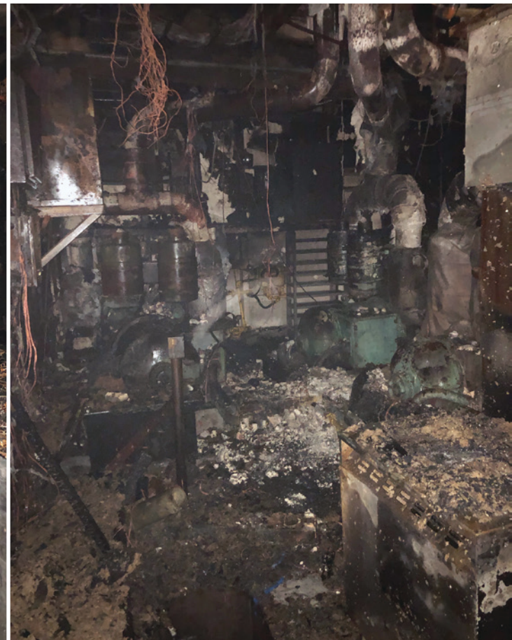
Figure 106. Fire damage to living quarters (left) and generator room (right). SOURCE: COAST GUARD
