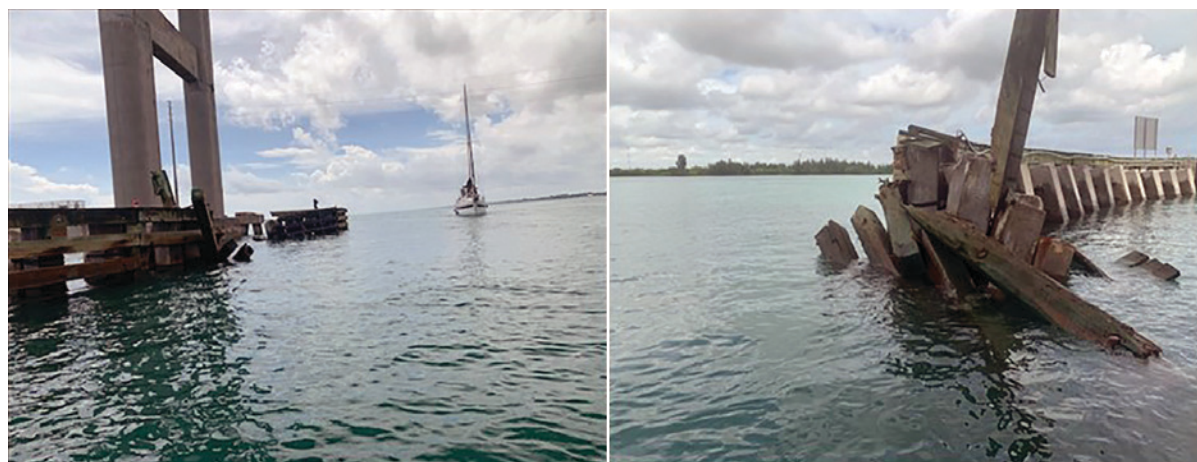
Figure 74. Postaccident damage to the eastern fendering of the bridge looking to the south (left) and to the north (right). SOURCE: COAST GUARD
