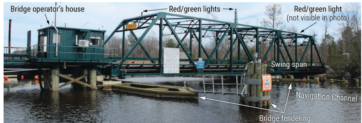
Figure 66. Centerville Turnpike Bridge in the closed position. BACKGROUND SOURCE: CITY OF CHESAPEAKE
