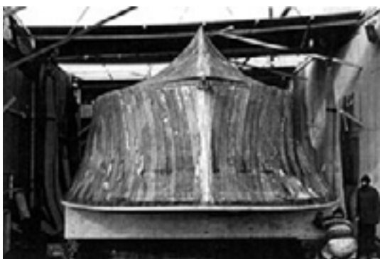
Inverted for outer bottom work
