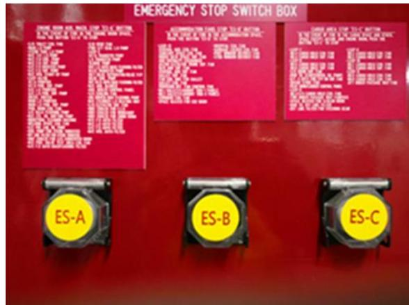
Figure 6 - Emergency Stop Switch box of a sister ship
