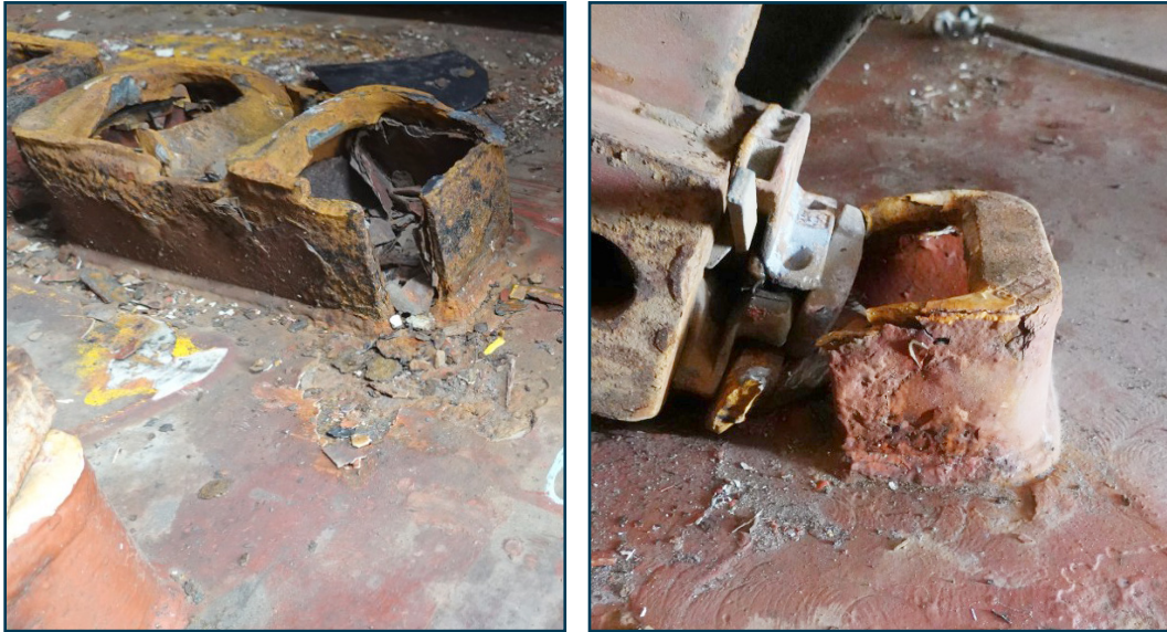
Figures 49 and 50: Example of socket fractures – bay 66 and 38 Source: Maersk A/S
