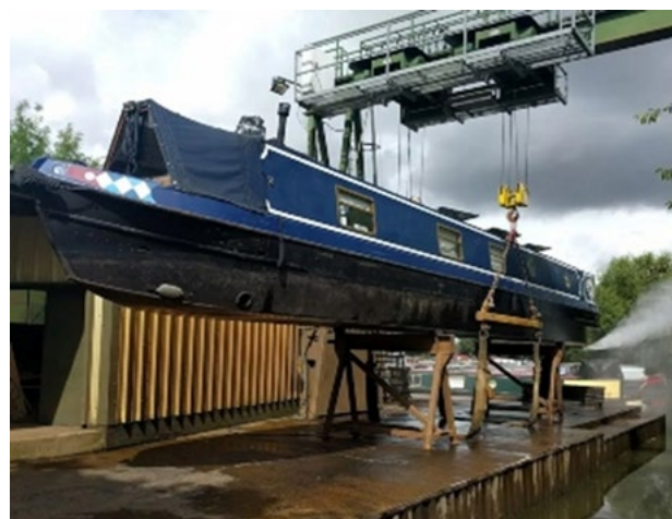
Work in progress at Debdale Wharf Marina
