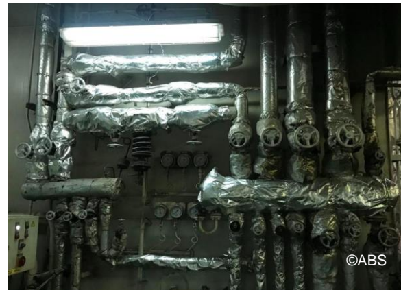
Missing pipe insulation restored
