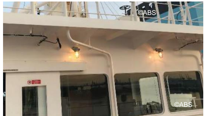
Operational test of emergency lights after repair
