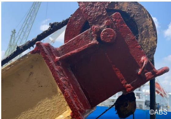
Rescue boat davit found corroded
