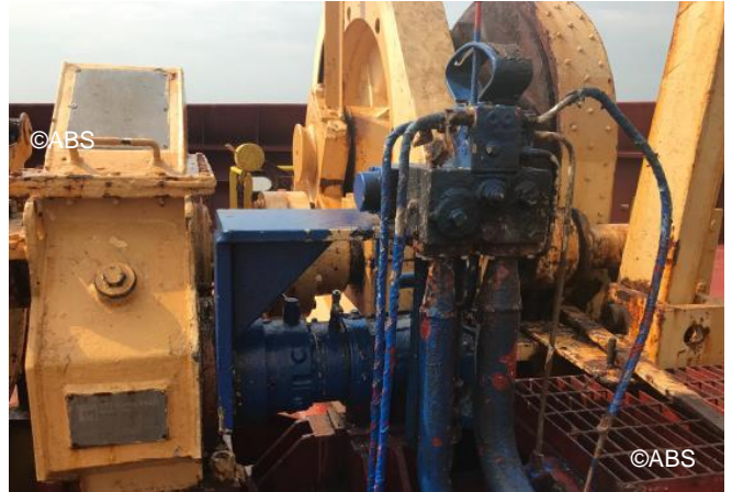
Damaged hydraulic motor for mooring winch replaced
