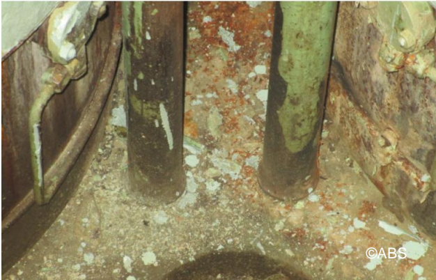
Main engine cylinder cooling water leak
