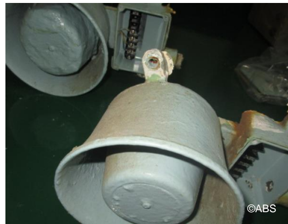
Public address speakers not functioning
