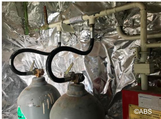
Paint store CO 2 hoses replaced
