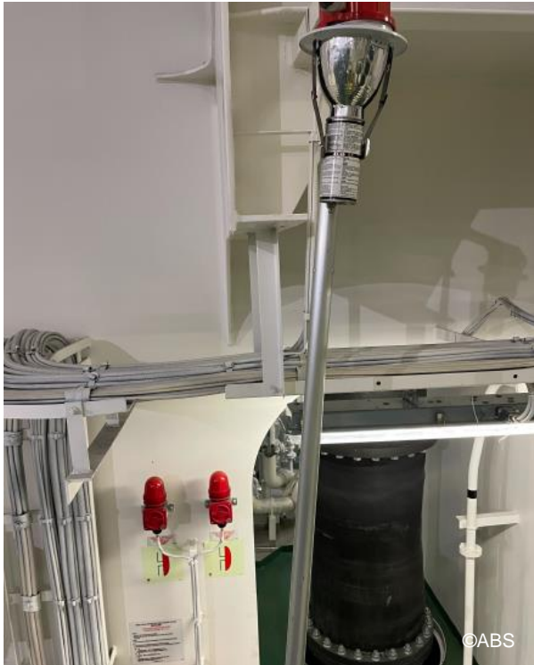
Testing engine room fire detector after repair
