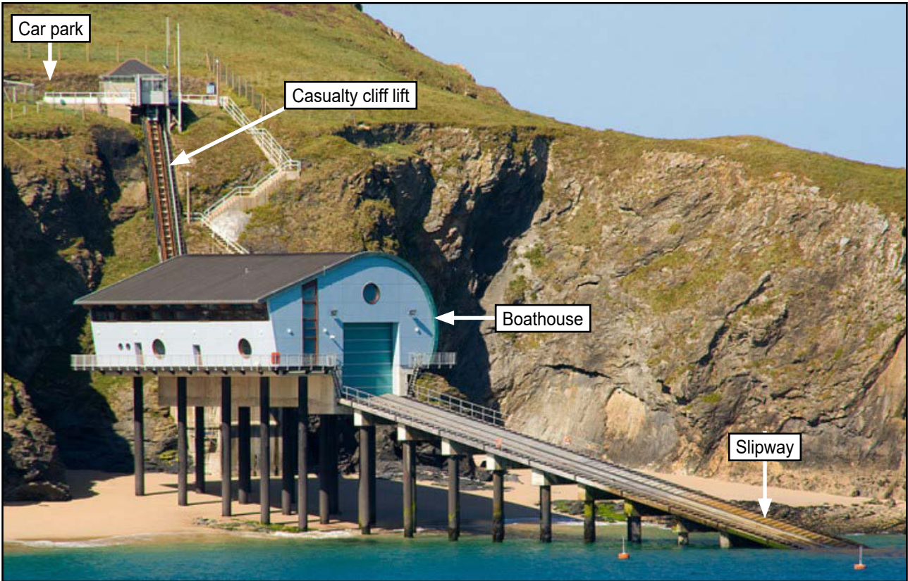
Figure 5: Padstow Lifeboat Station
