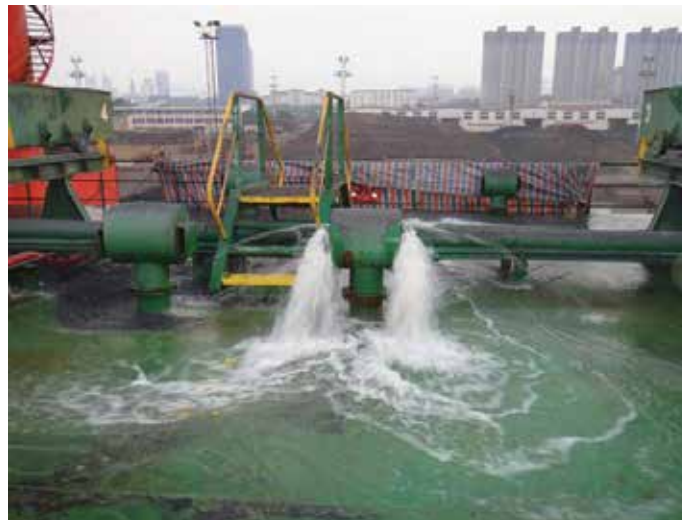
Figure 2.8 | Ballast tank hydro-testing.
