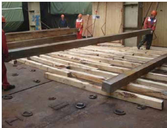
Figure 4.6 | Dunnage being prepared for carrying heavy cargo.
