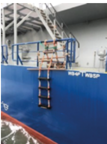
Sideway shuffle again – how strong is the railing?
