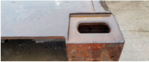
Chamfer on the lifting socket can be clearly seen.
