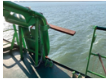
Non-compliant (by design) pilot ladder winch reel, spreader obstructing entrance after the sideways dive.
