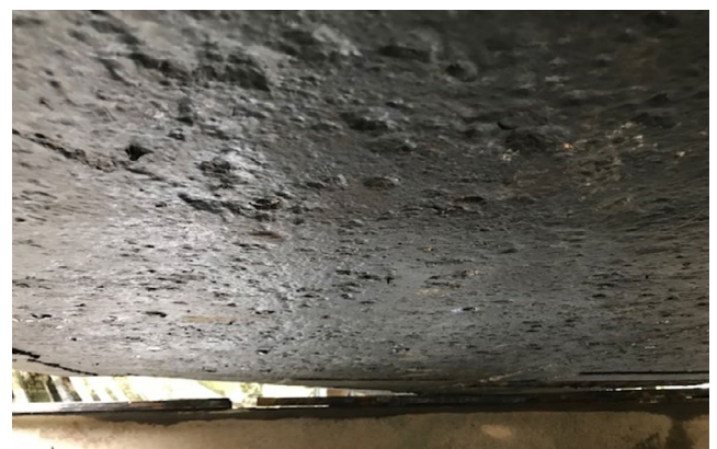
Photograph 1. Galvanic pitting on the unpainted bottom of a Dutch Barge
