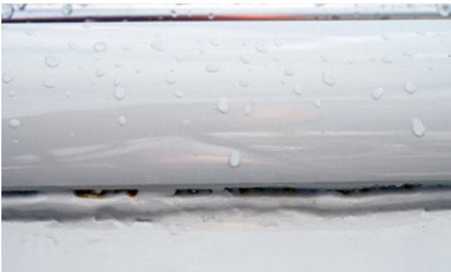
Fig 6. Poor welding beneath a rubbing strake on another vessel.
