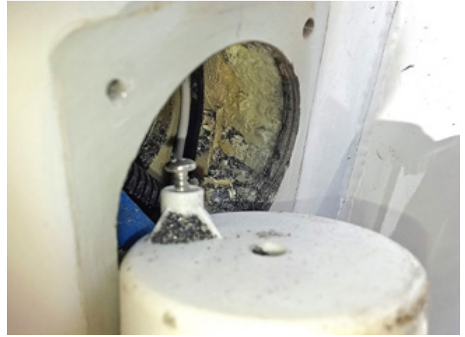
Fig 5. Unprimed steel and loose swarf behind an external electrical fitting.
