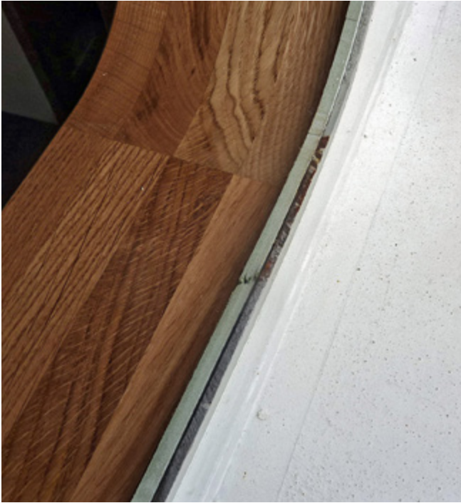
Fig 4. Unprimed and rusting steelwork around window cut outs.
