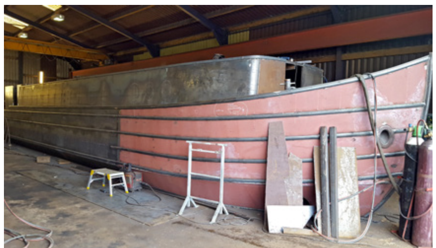
Fig 2. The forward section of this Dutch Barge hull was being fabricated in pre-primed, shot blasted steel whilst the remainder was fabricated in black steel. Note the lack of access to the flat of bottom and the lack of water freeing ports in the solid steel bulwarks.
