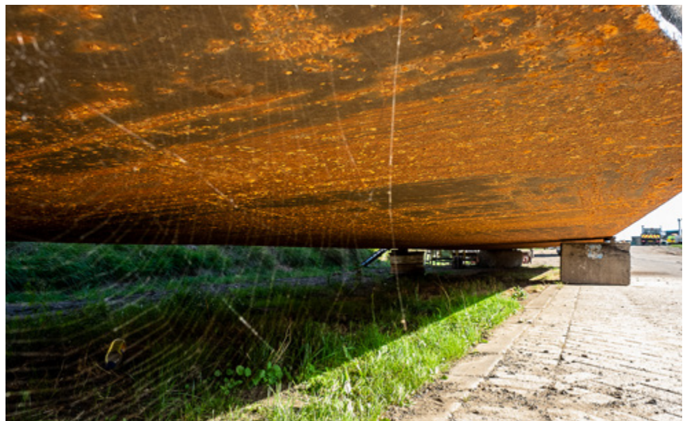
Fig 8. The flat of bottom was unpainted black steel and even in fresh water had been corroding freely.
