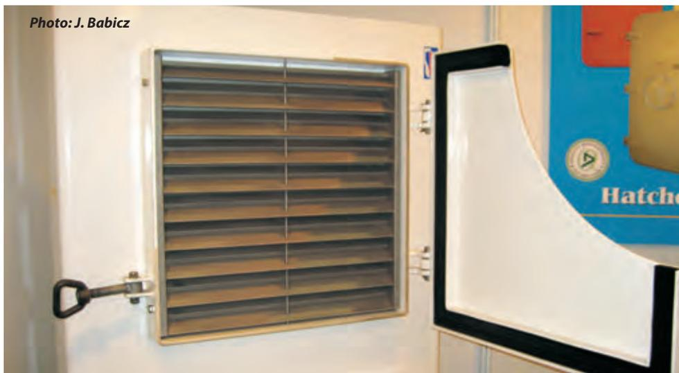
**Jalousie** – A shutter or cover with louvers. It provides ventilation while restricting the entry of rain and wind.
