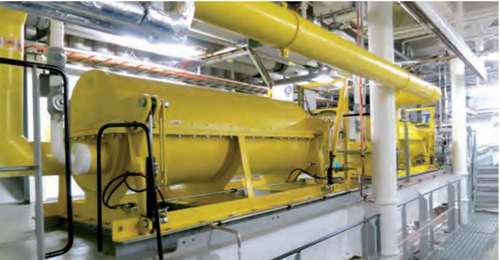
**Wärtsilä Gas Valve Unit Enclosed Design (GVU-ED™) installed directly in the Engine Room**
