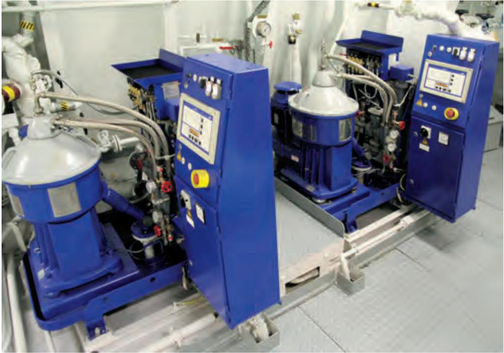
*Separation system modules from Alfa-Laval*
