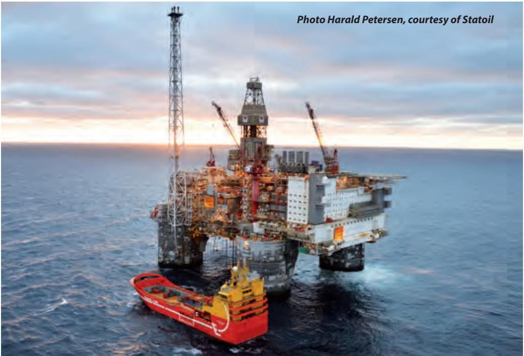
*Gravity Base Structure on the Heidrun field*
