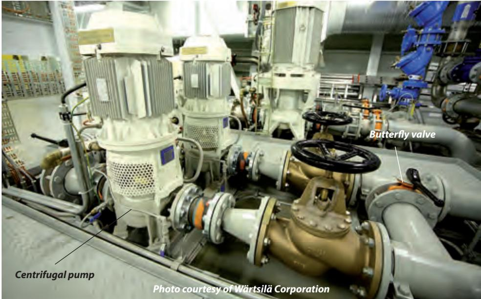
**Centrifugal pump** – It develops its pressure as a result of centrifugal force. Liquid enters the centre of the impeller and flows radially out between vanes. Its velocity being increased by the impeller rotation. It escapes through a discharge pipe at the circumference of the casing.
