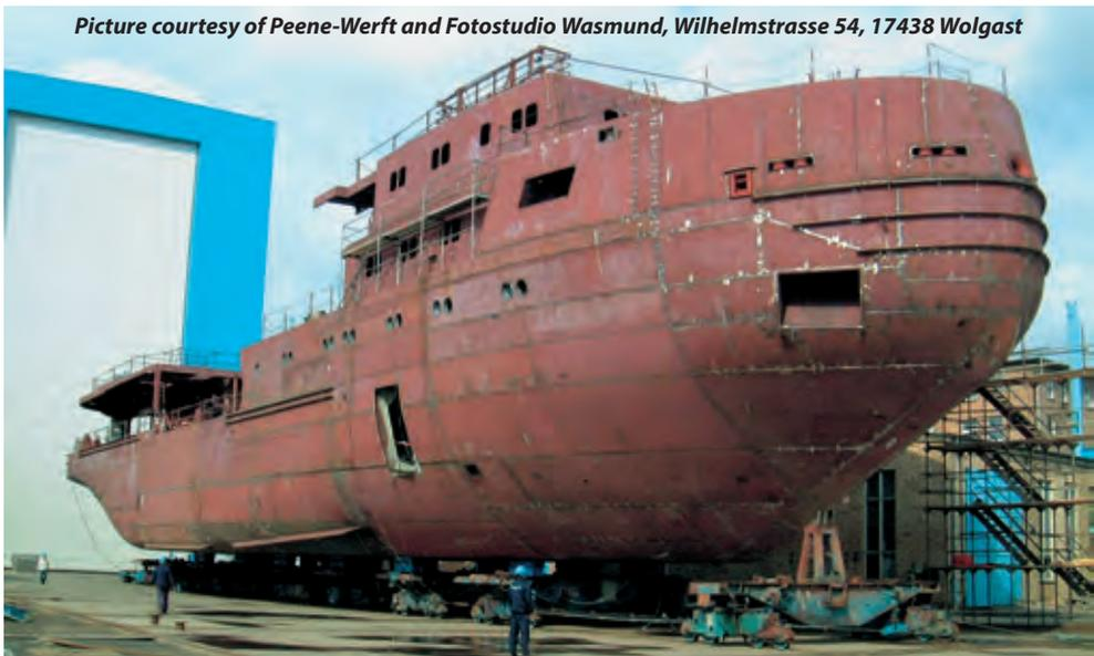
*Hull of the oil spill response vessel ARKONA built by PEENE-WERFT
