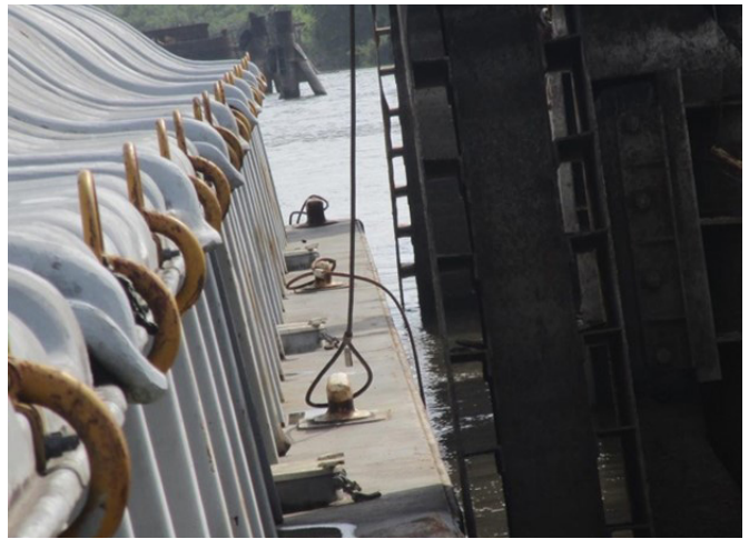
Figure 11B | Barge Fleet Moorings in a Rising River
