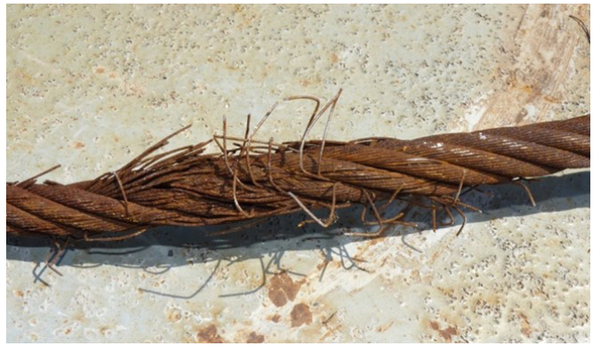
Figure 7B | Wire ropes in poor condition
