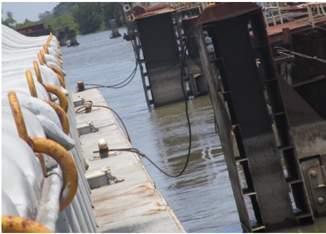
Figure 11A | Barge Fleet Moorings in a Rising River
