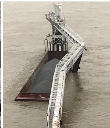
Figure 5 | Runaway barge leaning on a structure
