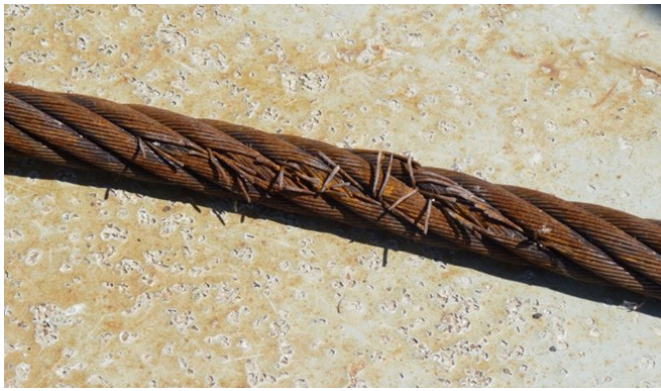
Figure 7A | Wire ropes in poor condition
