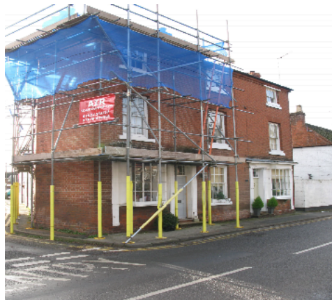
Vertical uprights and bracing
