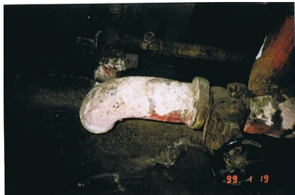
Damaged asbestos thermal insulation on pipework
