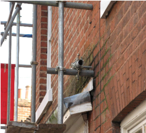
Secured by ties
