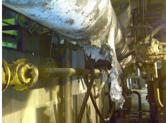
Damaged asbestos thermal insulation
