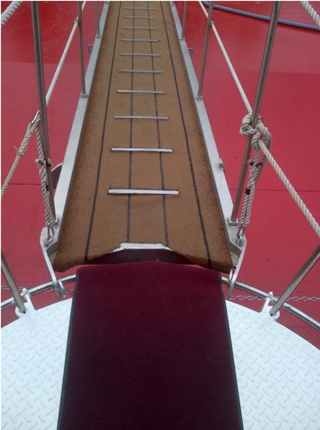
Example D: Gap between gangway and platform (trip hazard).
