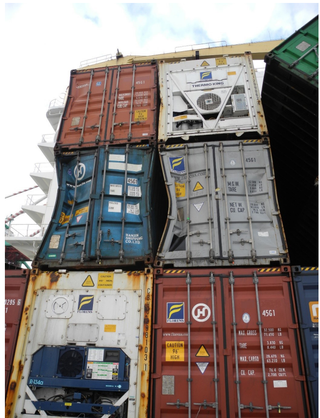
Figure 43: Damaged container showing corner post compression
