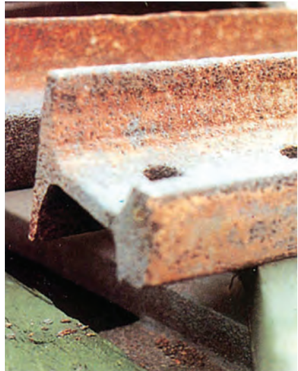
Fig. 12. Rails. Surface-condition clause: rust with pitting
