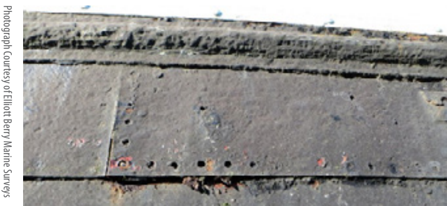
Photograph 2 - Sheerstrake Plate blown off the Ship's Side by Crevice Corrosion between the Plate and the Frames and on the Landing Strake Seam
