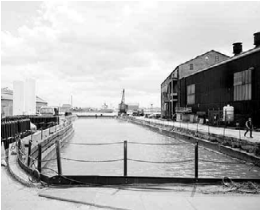
Blackwall Yard No 2 dry dock. The last on the London river and now a listed building.
