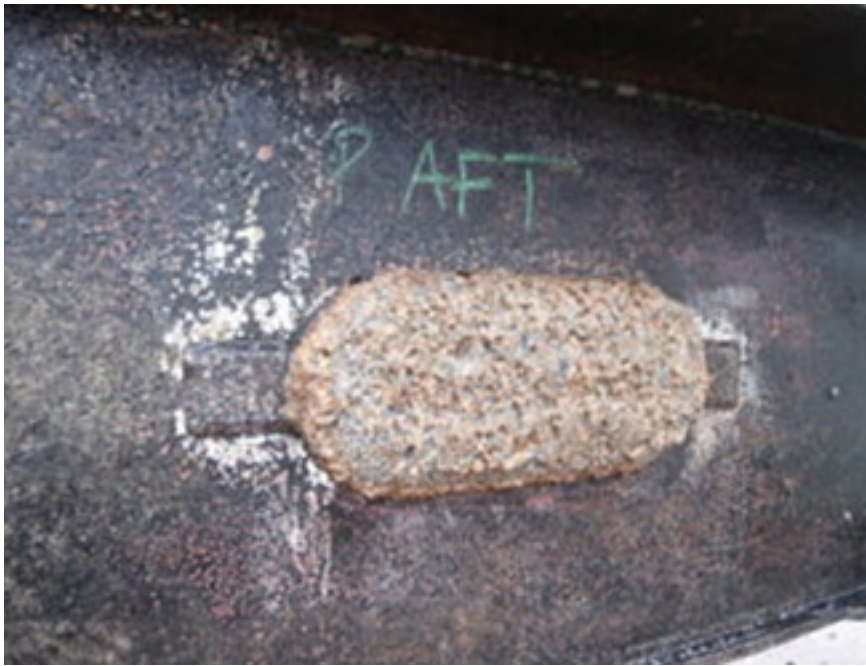
Part wasted magnesium anode with deep irregular pits
